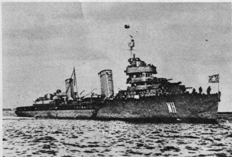
LENINGRAD CLASS DD's are big, fast ships (2,900 tons, 36 knots), poor sea boats. Leningrad ( above ) has gun between bridge and stack.
